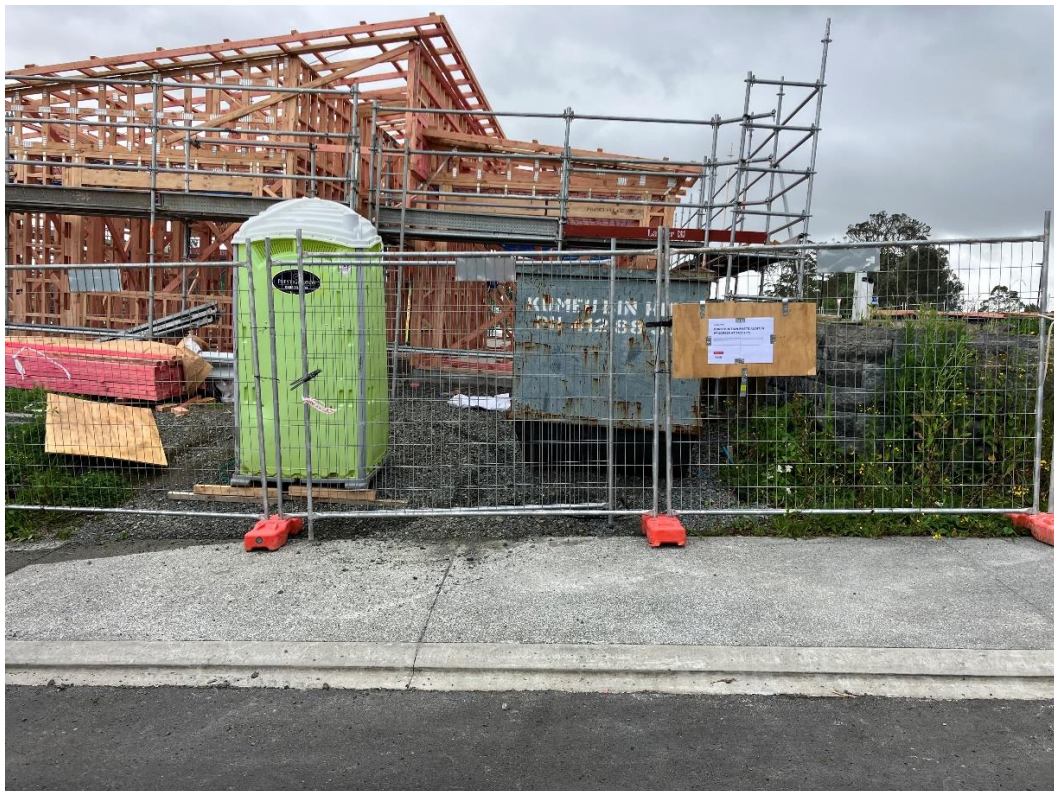
FIGURE 1: SITE SECURITY FENCING.
