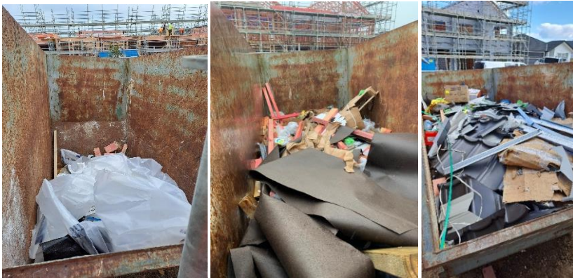
FIGURE 3: EXAMPLES OF SKIPS FILLING UP ON SITE.
