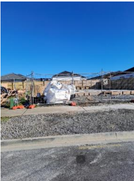
FIGURE 9 EPS WASTE FROM THE FLOOR INSTALLATION AWAITING COLLECTION FOR RECYCLING
