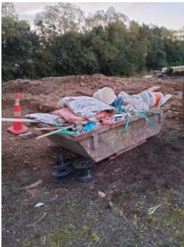
FIGURE 7 WASTE PACKED FOR DISPOSAL
