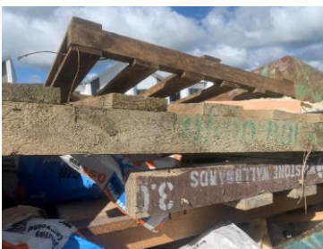
FIGURE 11 DEPOSITED GIB PALLET PLACED IN A SKIP.
