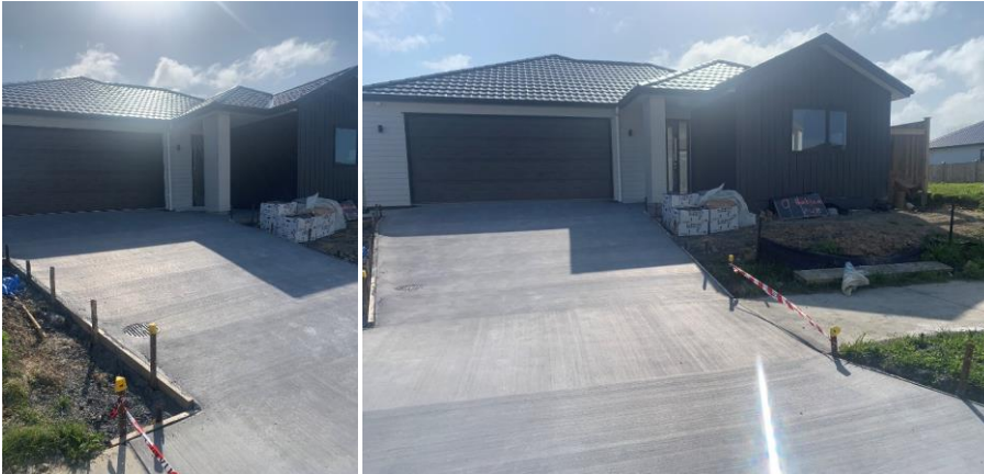
FIGURE 12 CONCRETE DRIVEWAY WITHIN THE FOOTPATH CUT OUT.
