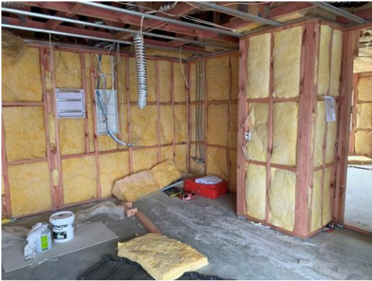
FIGURE 14 INSULATING MATERIAL DURING INSTALLATION.
