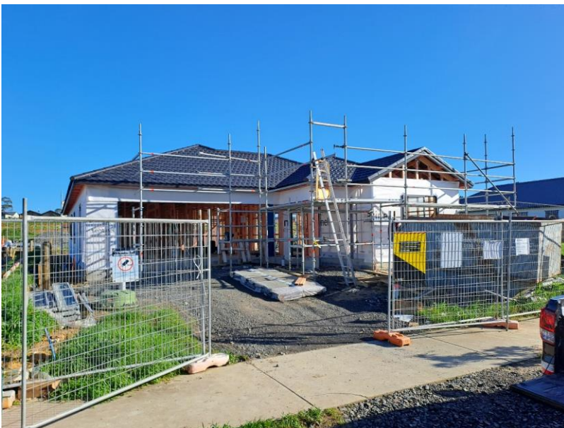
FIGURE 2 SITE SECURITY FENCING
