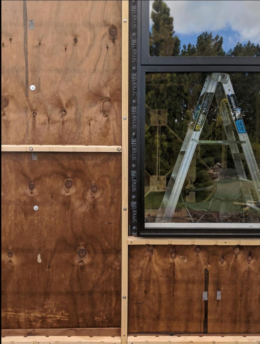
*T-Slot rebated groove in profiled timber cavity batten to receive intermediate bracket.*
